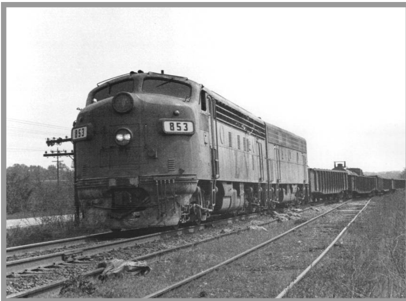
L&N F7A 853 and an unidentified B unit works the IC interchange at Nortonville, KY on May 5th, 1973. This tired old warrior will be off the roster in another 24 months after 24
